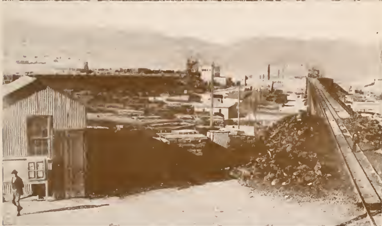
Curanilahue Coal Mine, Arauco Province. Dulcinea Copper Mine, Copiapó Province. Chuquicamata Copper Mine, Antofagasta Province.
